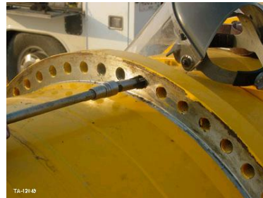
CLEANING PAINT AND RUST PRIOR TO TORQUING
